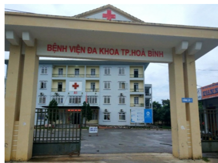
General hospital of Hoa Binh City, Vietnam.
