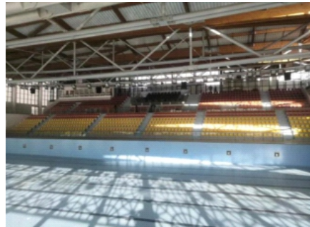
Swimming Pool Center, Algeria.
